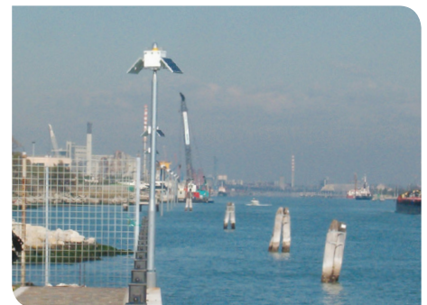
SL-125-C lanterns installed at marina, Venice, Italy
